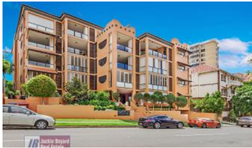
34 Moray Street, New Farm
